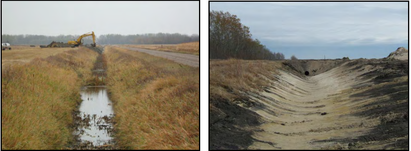
Permitted work – ditch cleaning and culvert installation
