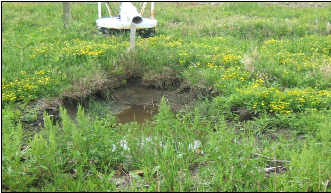
Erosion from a tile line pump that needs to be fixed in Project # 119
