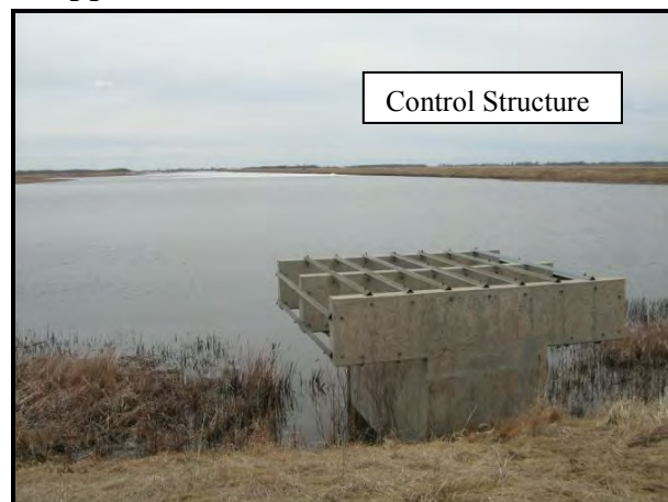
BR #6 – Impoundment, Polk County Upper Burnham Creek & CD #140
