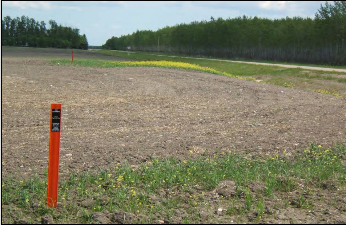
Right-of-way violation of grass buffer strip on Project # 117
