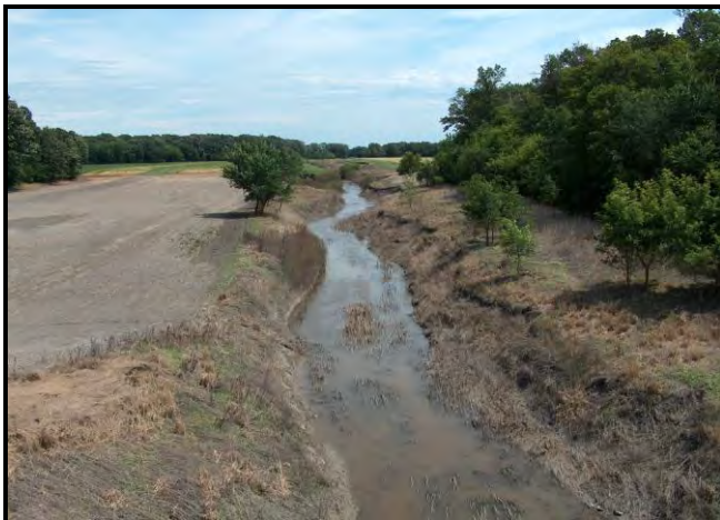
Looking East before construction (CSAH #64)
