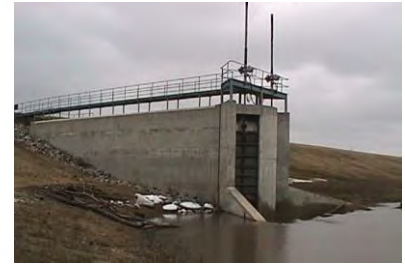
Principal outlet structure hydraulic gate operation
