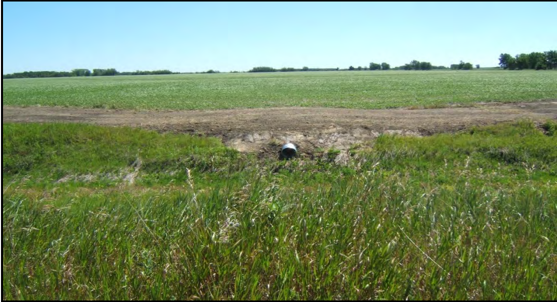
Side inlet pipe in RLWD Ditch 3
