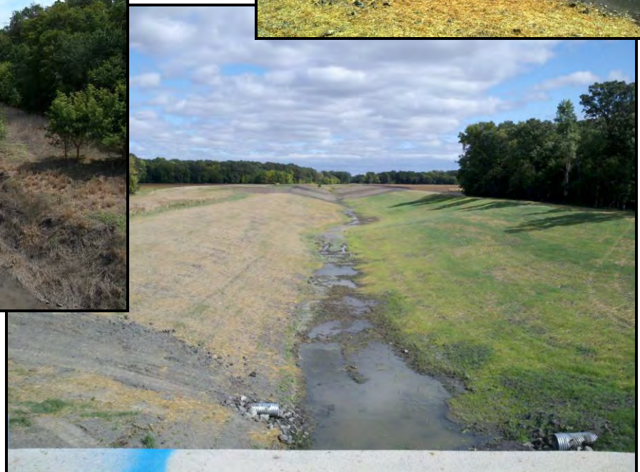
Looking East after construction (CSAH #64)
