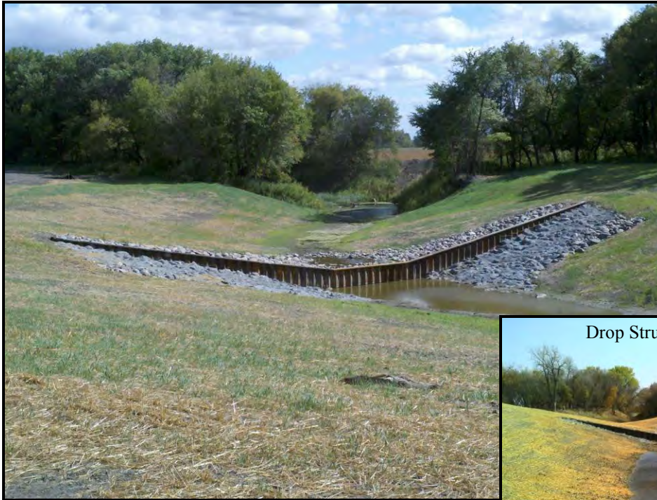
Drop Structure at Station 15+50
