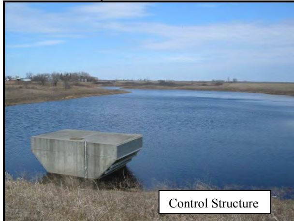
Baird Beyer Dam, Red Lake County Tributary to the Black River
