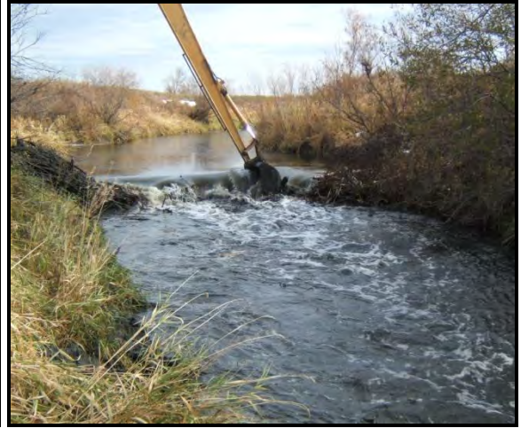
Removing beaver dam from Ditch 83
