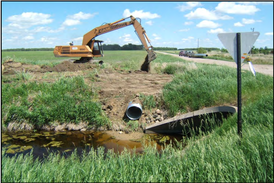
One of many side water inlet pipes being installed in RLWD Ditch 7
