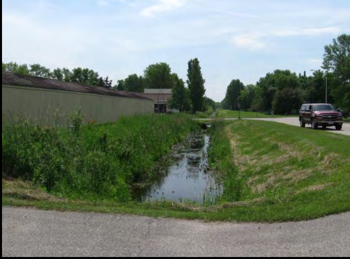
Edgewood Drive Before Construction
