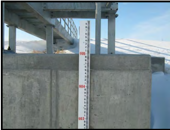
Typical staff gage at structure
