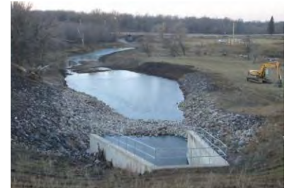
Looking downstream from outlet structure
