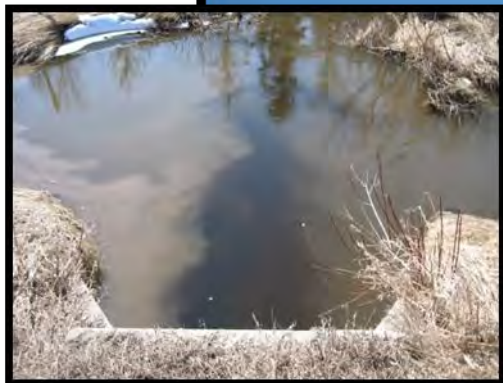
Above: Sediment plumes in Clearbrook from stormwater runoff.
